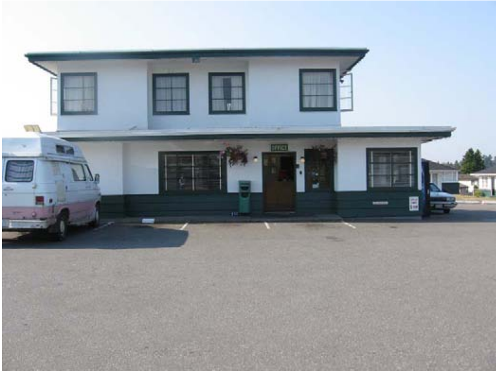
Fig. 3 Administrative Office building
