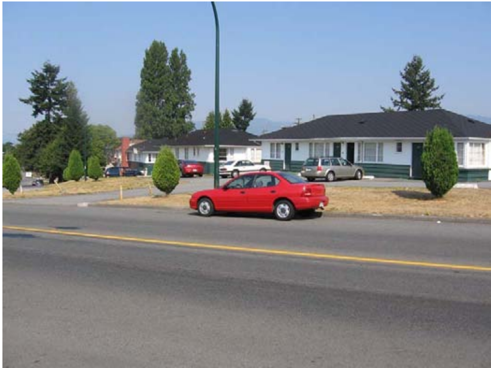
Fig. 11 Southern edge of Second Phase bungalows looking northwest
