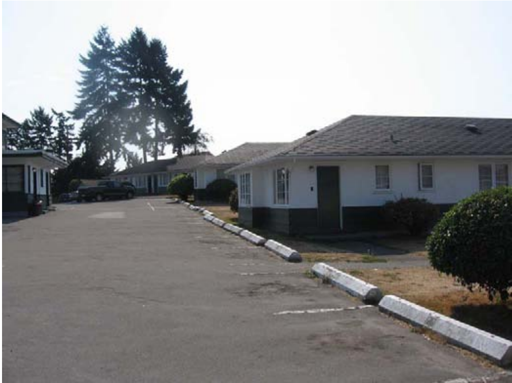
Fig. 7 Second Phase bungalows south of administration building
