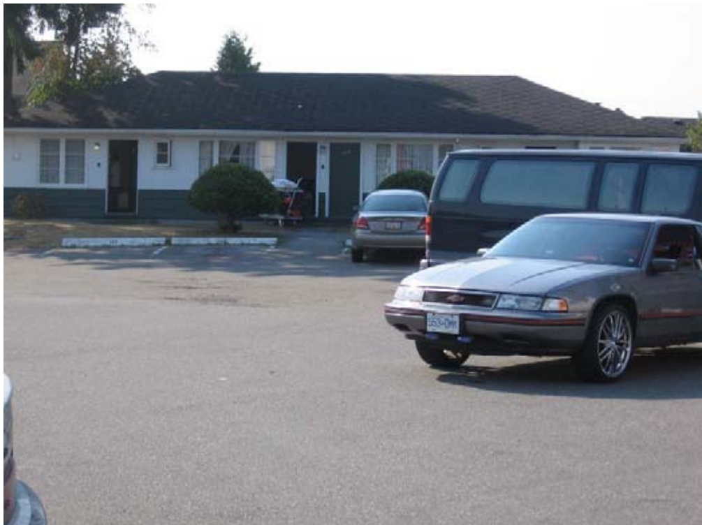
Fig. 8 Second Phase bungalows south of administration building
